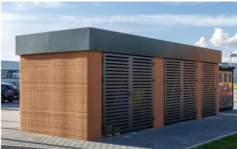
First buildnig in Poland printed on site
