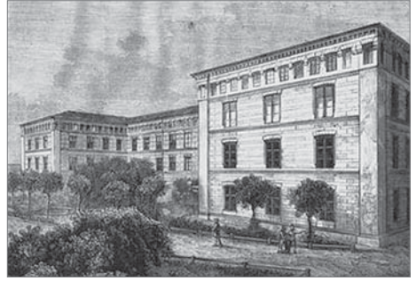
The first building of the Tsar Nicholas II Polytechnic Institute of Warsaw on Marszałkowska Street
